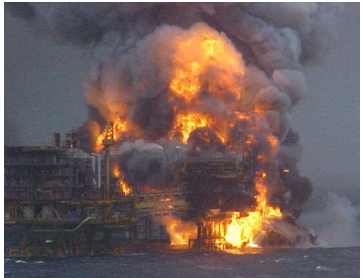
BOMBAY HIGH NORTH oil rig on fire The cook cut his finger and was hoisted to the rig, the boat hit the gas riser and caused the fire
