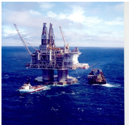
(File photo – Hibernia Platform, a Great Lakes self-unloader pumping ballast into the outer shell of the Platform)
